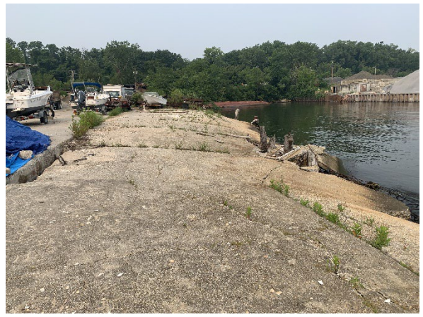
From the northeast corner of the concrete platform, facing west.
