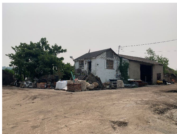
One-story building on the Subject Property.
