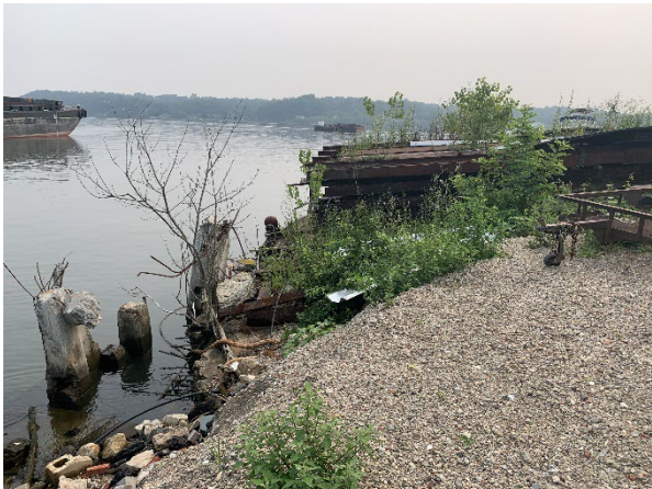
From the northern portion of the concrete platform, facing east towards Hempstead Harbor.
