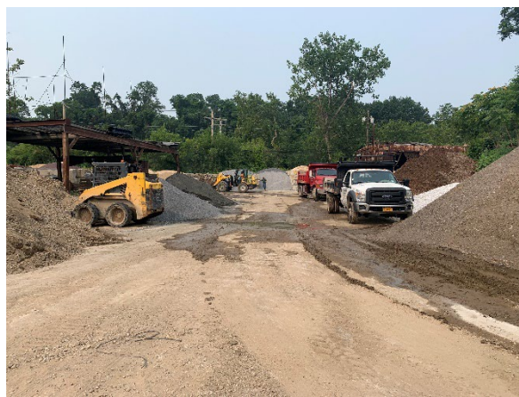
View of the interior of the Subject Property.
