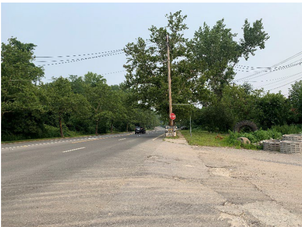
West Shore Road facing north.
