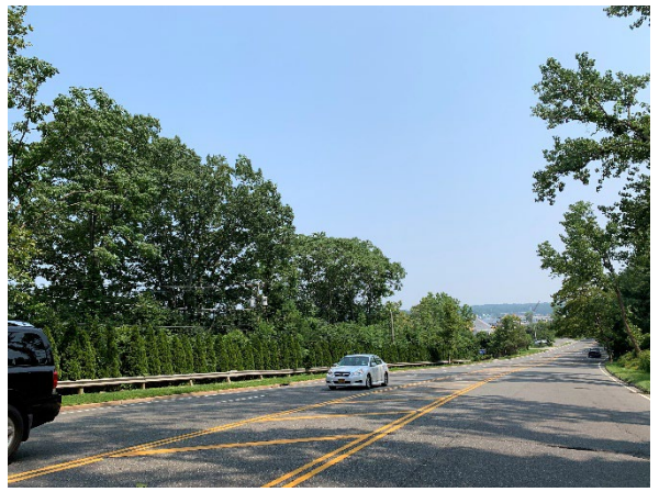
West Shore Road facing southeast.
