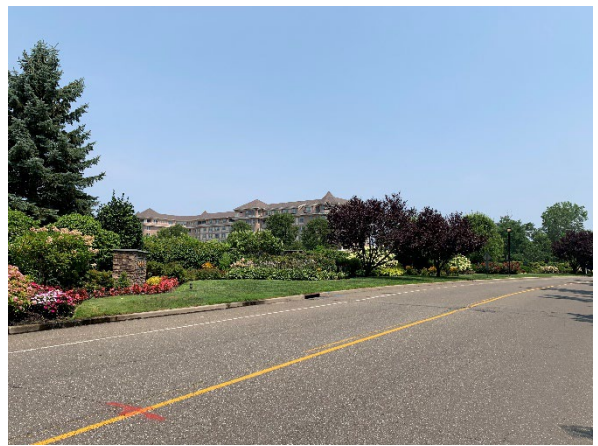
View of the six-story, Amsterdam at Harborside multi-family residential development, facing northeast.
