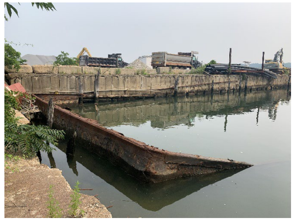
From near the northwest portion of the concrete platform, facing northeast.
