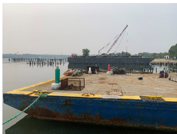
Representative view of the dock used in association with the gravel and sand storage, facing south.
