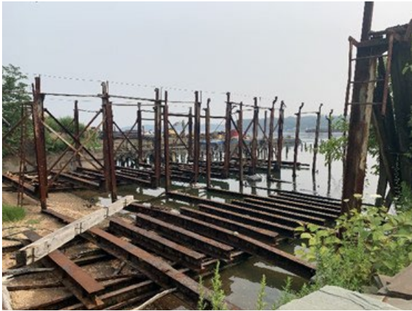
From near the existing concrete block building, facing northeast towards Hempstead Harbor.
