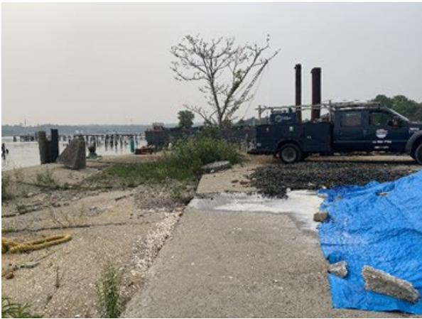
From the northeast portion of the concrete platform, facing south towards North Hempstead Beach Park.
