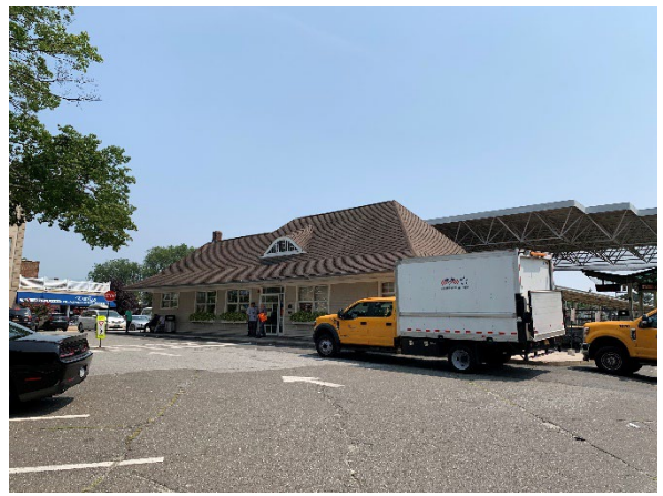
Port Washington Long Island Rail Road Station, facing southeast.
