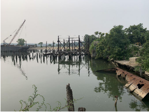
From the southwestern portion of the concrete platform, facing south towards North Hempstead Beach Park. A sunken barge is also visible.
